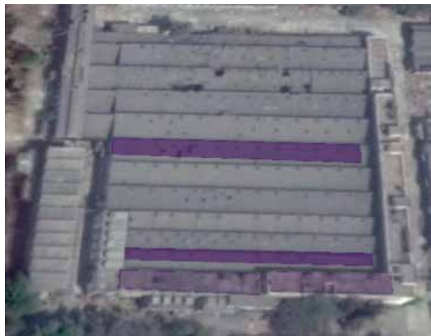
Figure 2.9: Shade free area of Tata Steel building library
