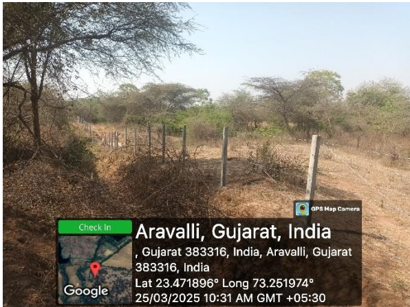
Barbed wire fencing
