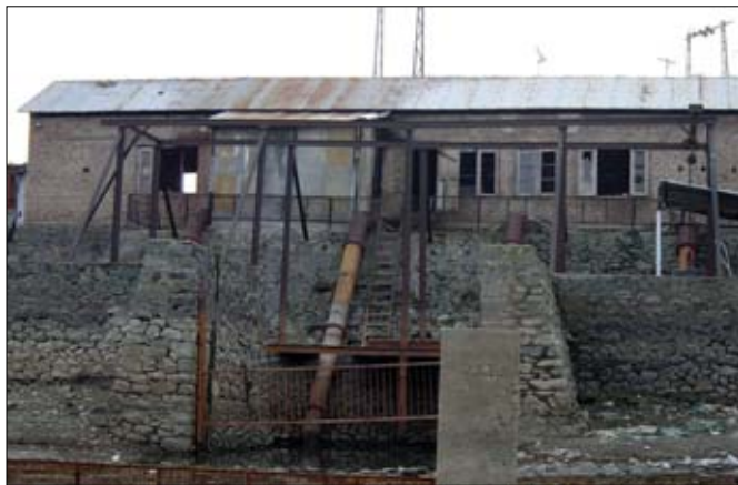
Water Lift Station at Watlab
